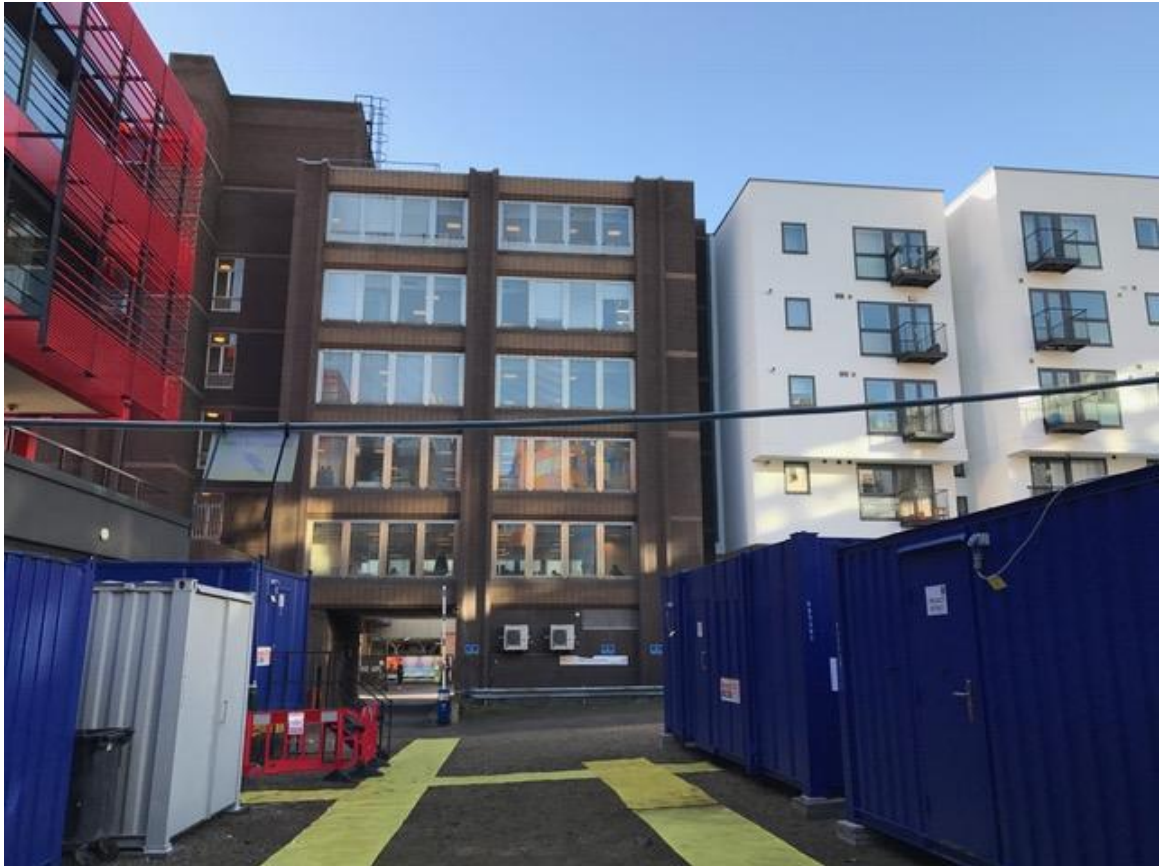
Image 2 – View from the site towards 6-storey office building fronting Turnmill Road.
